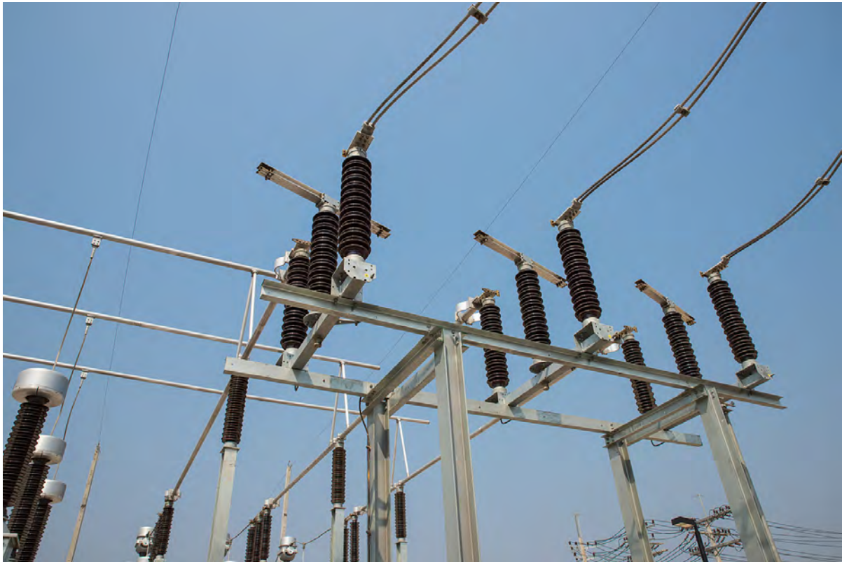
Figure 6: Pivoted, open isolators
